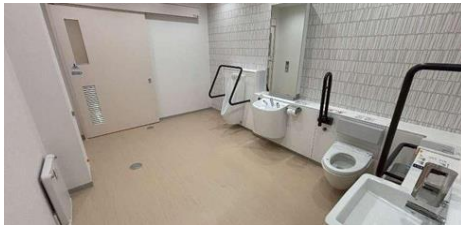
Adjusting the height of buttons and switches in ostomate-accessible restrooms to create a user-friendly design for everyone.
